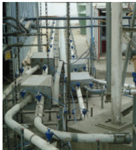
Boosters on two lines for cement pneumatic conveying.
