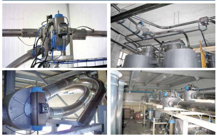
VAR Drum-Type Diverter Valves are essential components of all kinds of pneumatic conveying systems in those points where the material flow has to be diverted from one duct to another.
