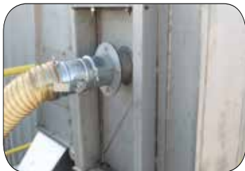
Dedusting nozzle on head section
